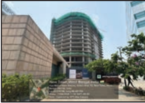
Under-Construction Commercial Block
