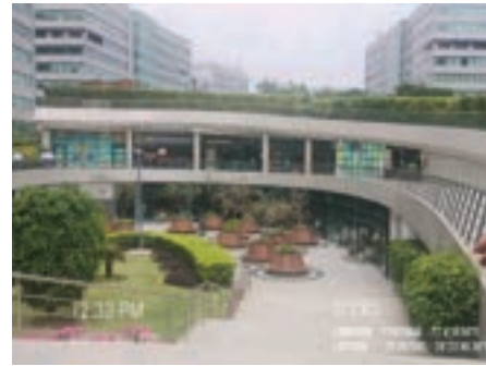
External View of Subject Property
