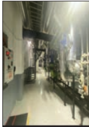
Internal View of Plant Room Tower 4, 5 & 6
