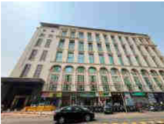
External View of Subject Property
