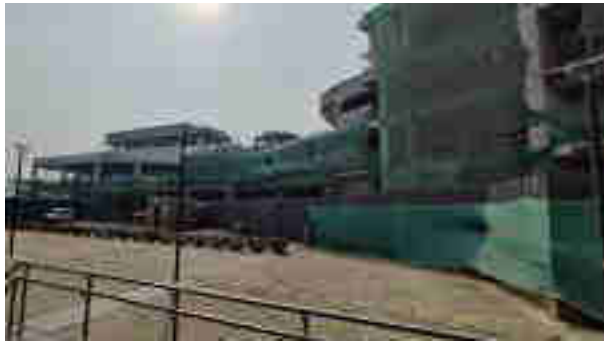
Under-Construction Commercial Block
