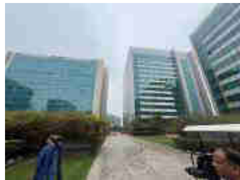
External View of Subject Property
