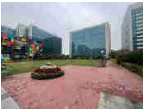
External View of Subject Property
