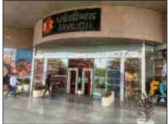
External View of Subject Property
