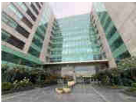
External View of Subject Property
