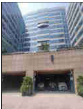
View of Tower 9
