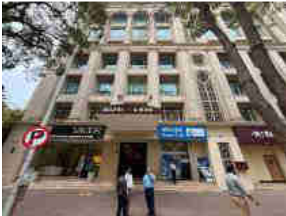
External View of Subject Property
