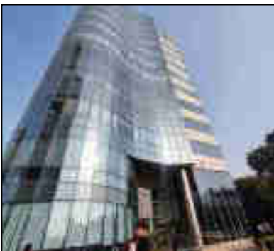
View of Block 1
