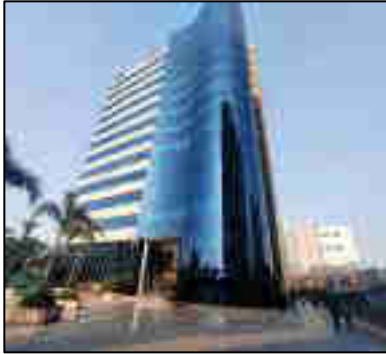
View of Block 3
