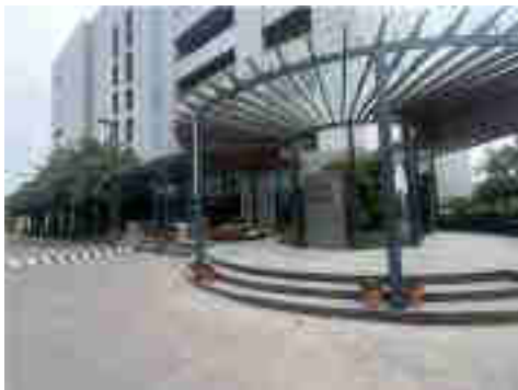
External View of Subject Property
