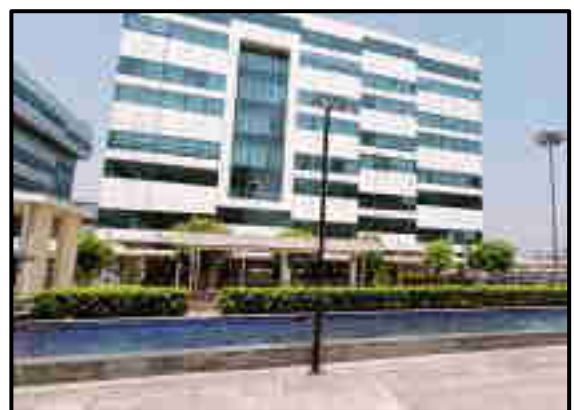
View of Tower G3
