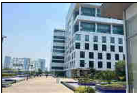
View of Tower G3 and C2
