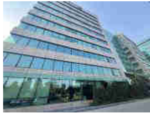
External View of Subject Property
