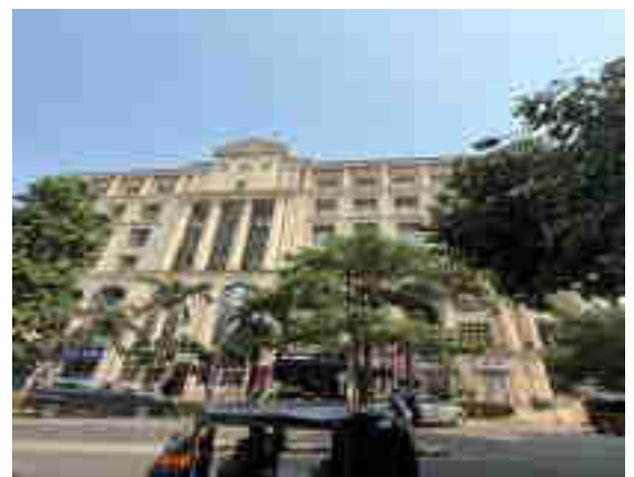
External View of Subject Property
