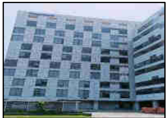
View of Tower C3
