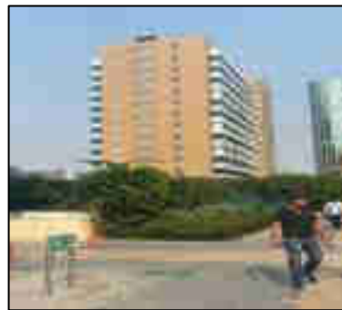
View of Block 6
