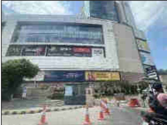
External View of Subject Property
