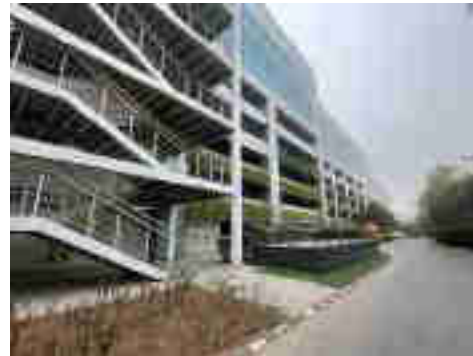
External View of Subject Property
