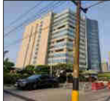
View of Block 2
