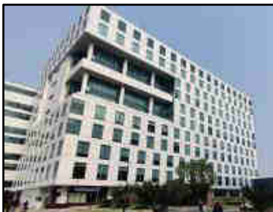
View of Tower C1
