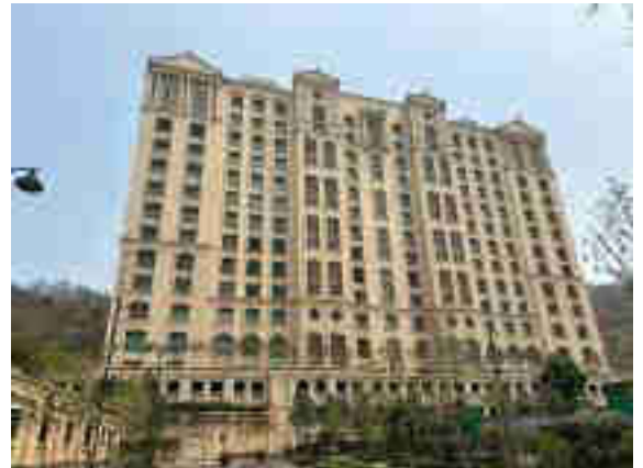
External View of Subject Property
