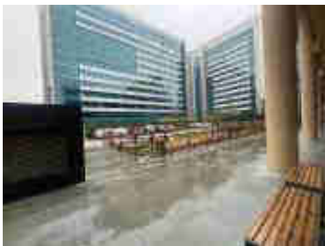
External View of Subject Property
