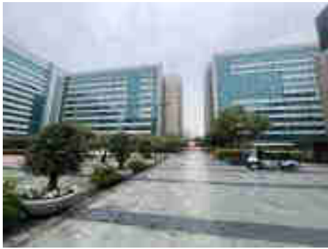
External View of Subject Property
