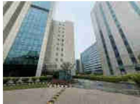
External View of Subject Property
