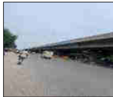
View of NH -48 (Secondary access road)
