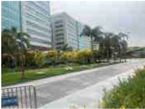
External View of Subject Property
