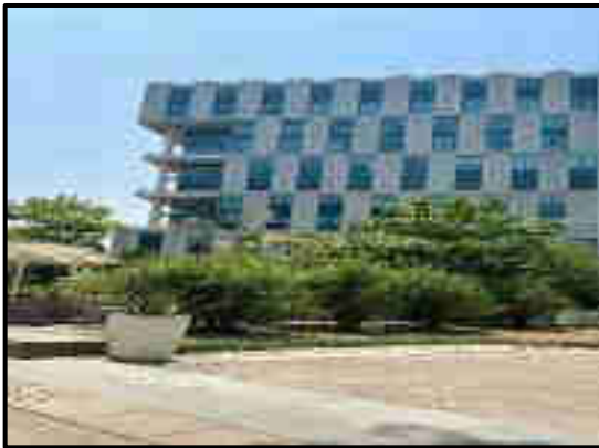
View of Tower A1
