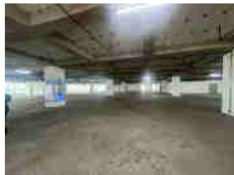
View of Basement of Subject Property
