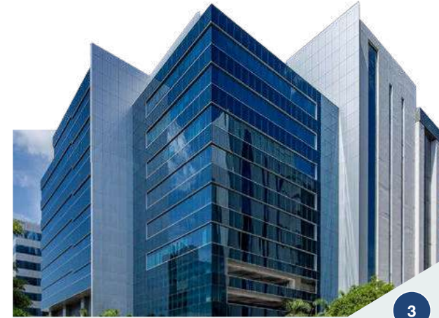
Commerzone Yewada and The Square Signature Business Chambers (Nagar Road), Pune
