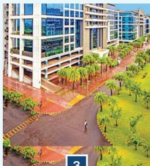
Mindspace Airoli (E) Mumbai Region Commerzone Yerwada and The Square Signature Business Chambers (Nagar Road) Pune Mindspace Pocharam Hyderabad
