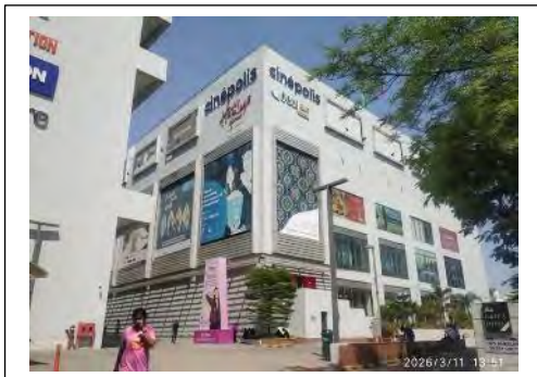
External view of the subject property
