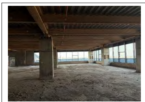
Internal view of the Subject Property
