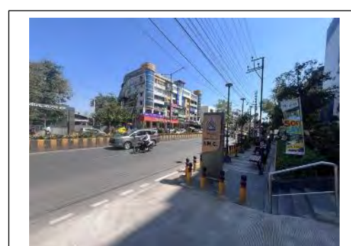
View of the primary access road
