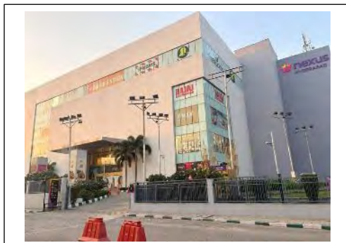
External view of the subject property
