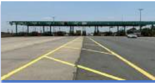
Chalageri Toll Plaza
