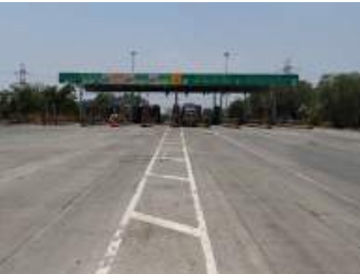
Boharipar Toll Plaza
