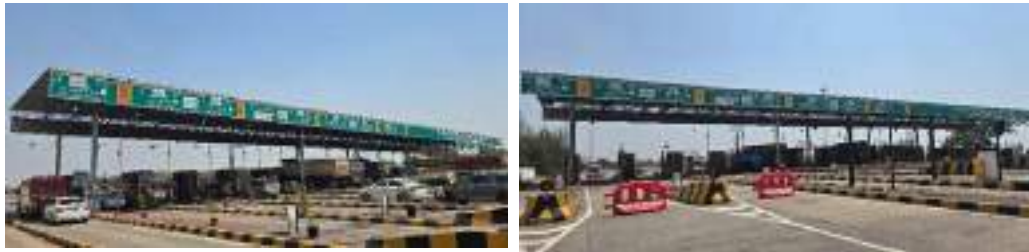
Bhojpuri Toll Plaza
