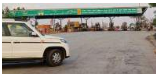
Dhaneshwar Toll Plaza
