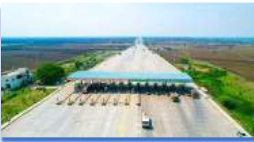
Bankapur Toll Plaza
