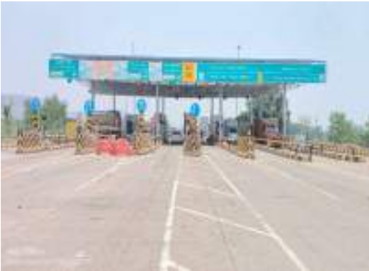
Kherwasani Toll Plaza
